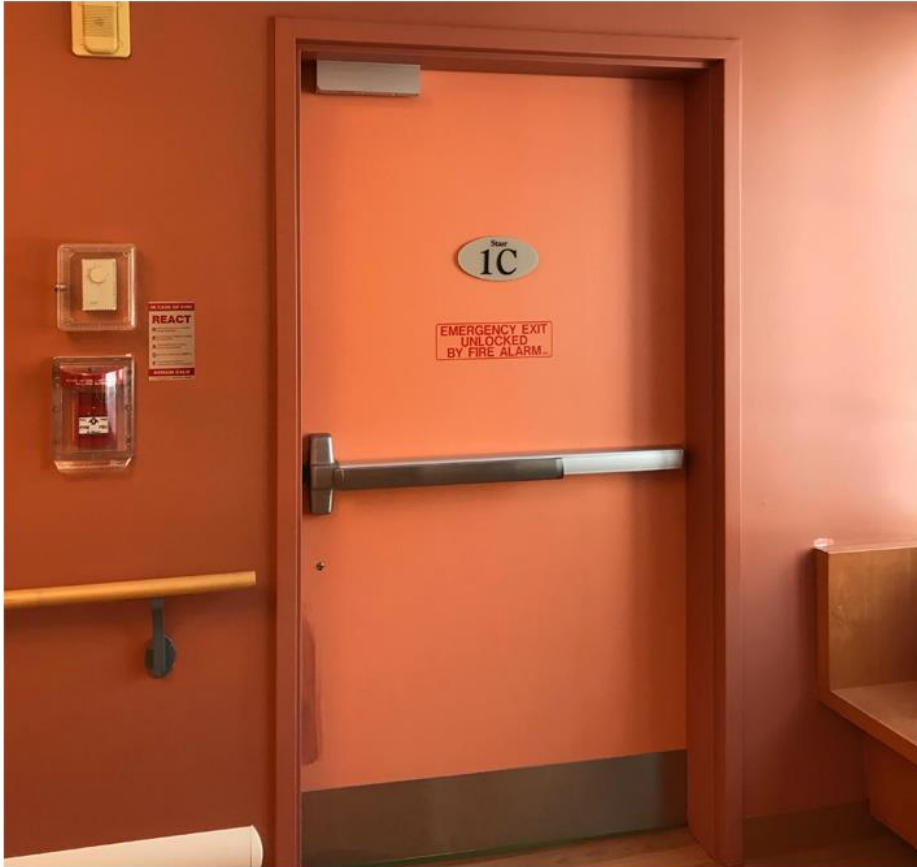
Stairwell Door Before
